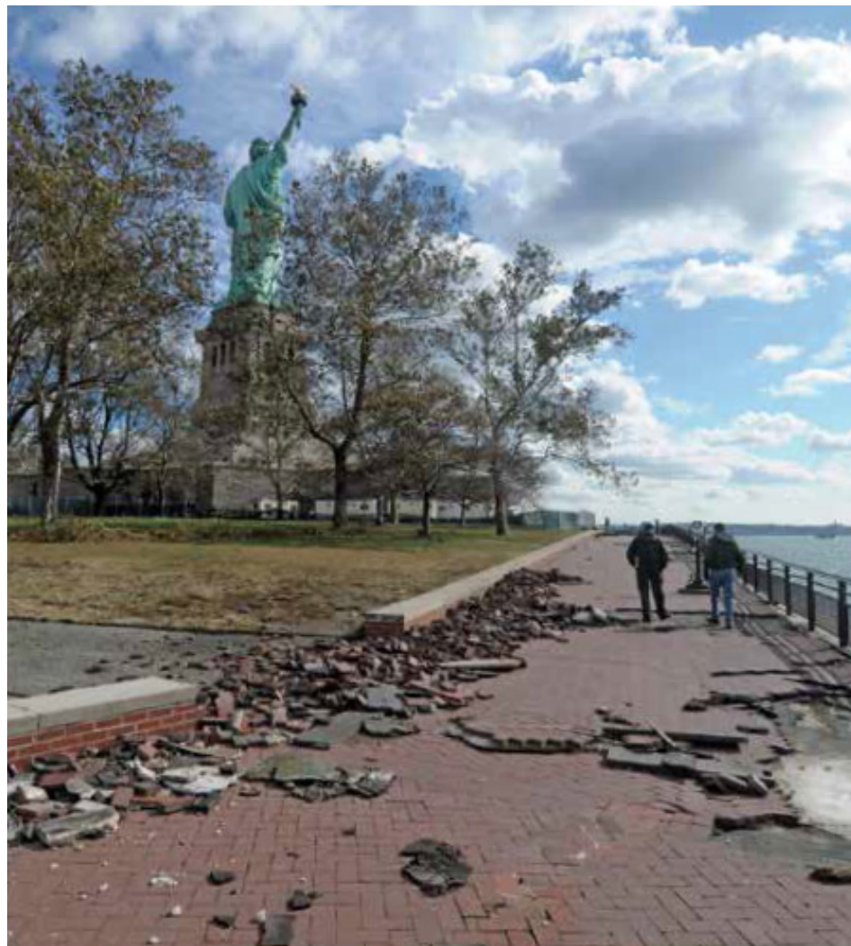
In 2012, Hurricane Sandy's storm surge damaged Liberty Island, closing it for eight months. Detail from "National Landmarks at Risk" (NPS/Daly).
